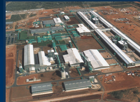
Mozambique Aluminium Smelter (Mozal)
